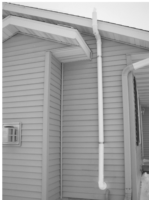
Figure 10 – Vent Line Installation
