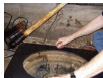
Crawlspace Sump Donut
