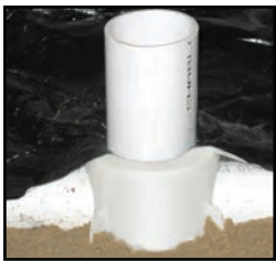
Cutaway view of Radon-T before sealing
