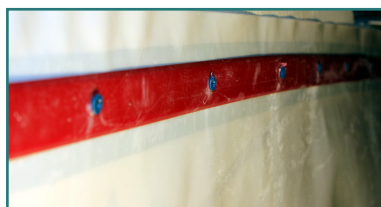
Stego® Term Bar: Typical Installation
