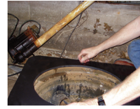
Crawlspace Sump Donut
