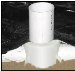
Cutaway view of Radon-T before sealing
