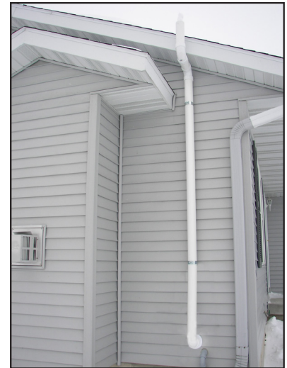
Figure 13 Vent Line Installation (3 inch)
