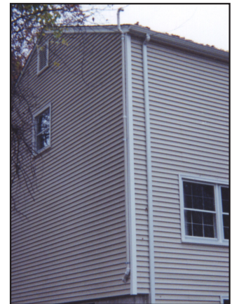
Figure 12 Vent Line Connection (2 Inch)
