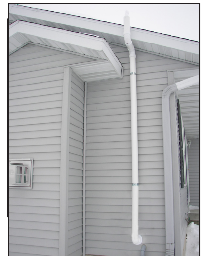
Figure 15 Air Intake Connection
