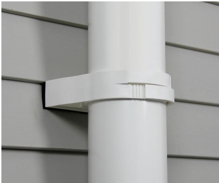
RadonAway fan motors are designed, built, and tested for noise and vibration. Any vibration that may occur after installation is often the result of the installation and not the fan itself. To further eliminate the potential for vibration, we match our pipe hangers with vibration-reducing dampeners, grommets and bushings.
